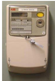
Panel-mounted solid-state electricity meter with remote current and voltage sensors, capable of being read, programmed remotely by modem and local infra-red.
