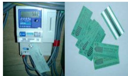
Prepayment meter and magnetic stripe tokens. Displays information and statistics such as current Tariff and remaining credit. Also has the provision to activate a small amount of emergency credit.
